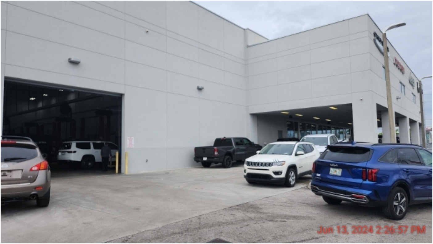
Photo 32: Entrance to the New Building.
