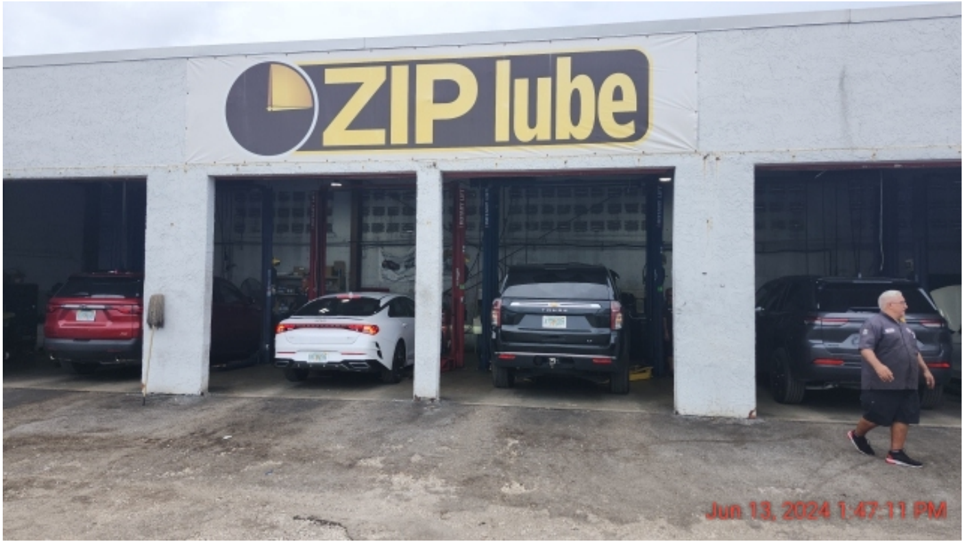
Photo 17: Entrance to the Quick Lube Shop.
