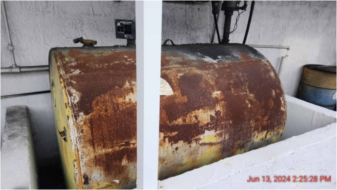
Photo 24: Used oil 500-gallon above ground tank outside the Western Shop.
