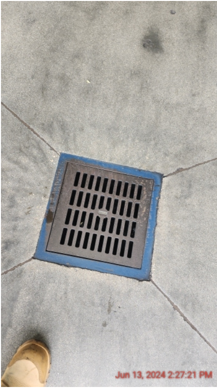
Photo 34: Floor drain to the new building.
