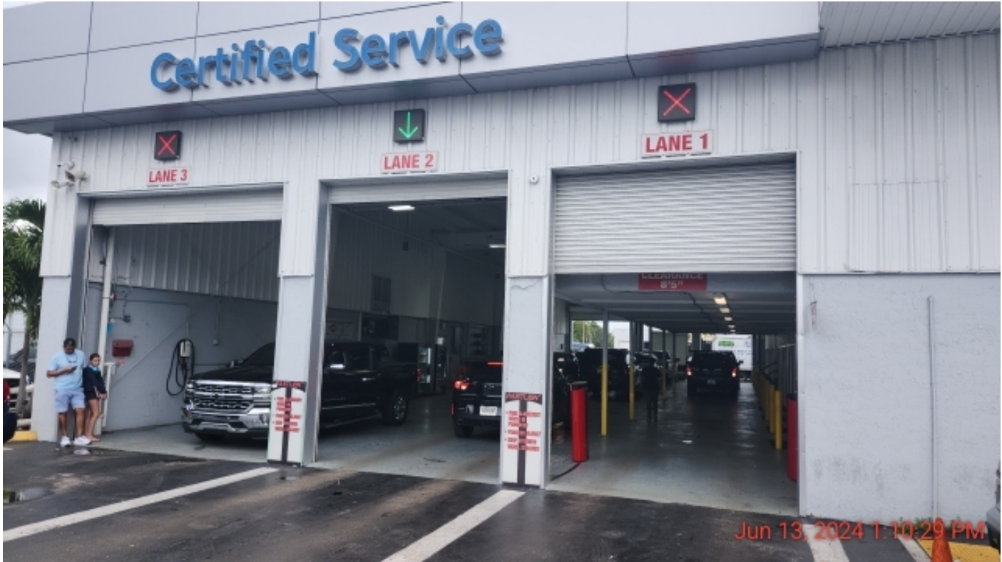
Photo 1: Overview of the front of the facility (service entrance)
