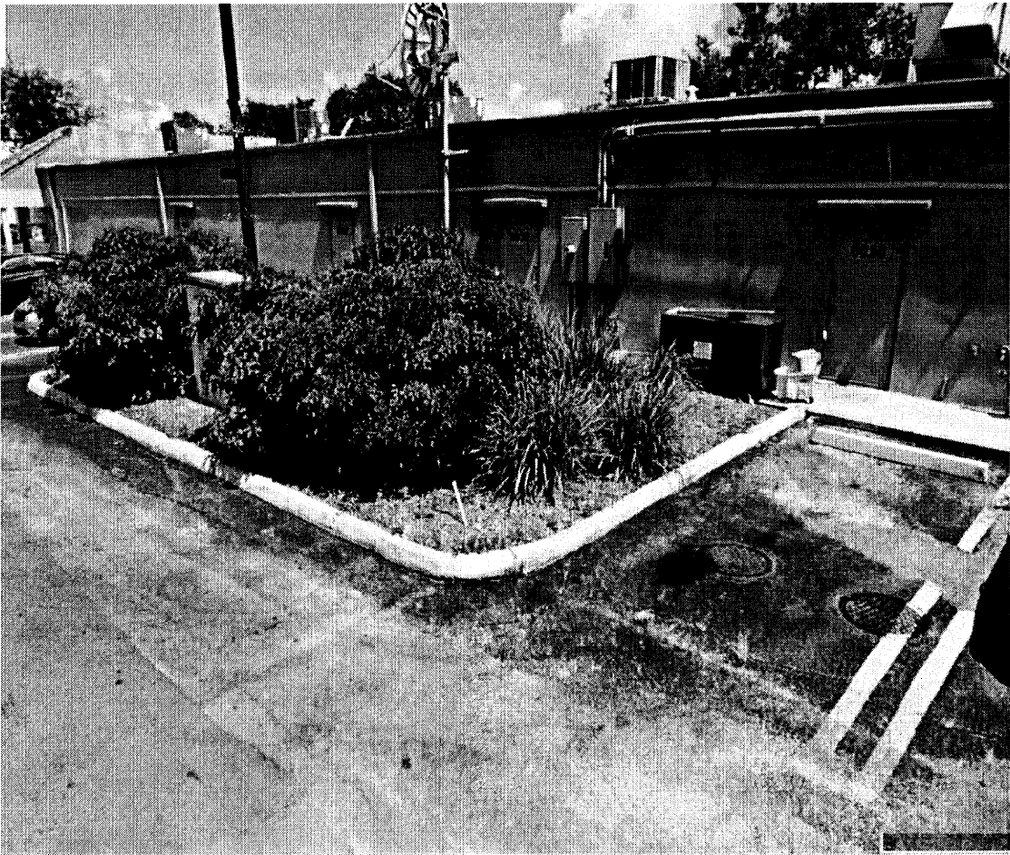
BACK EXIT DOOR TO PARKING VIEW
